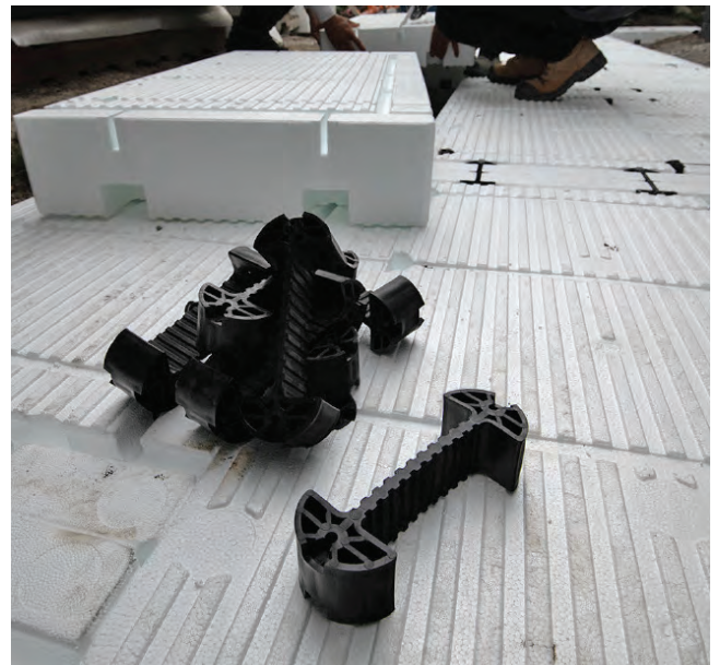
U-Core Connectors to lock units together
